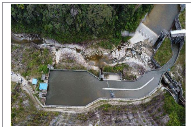
FIGURE 3: FOREBAY POND AND DAM AT PARMONANGAN PLANT
