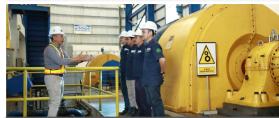
MHPP Parmonangan 2 (2 x 5 MW)
